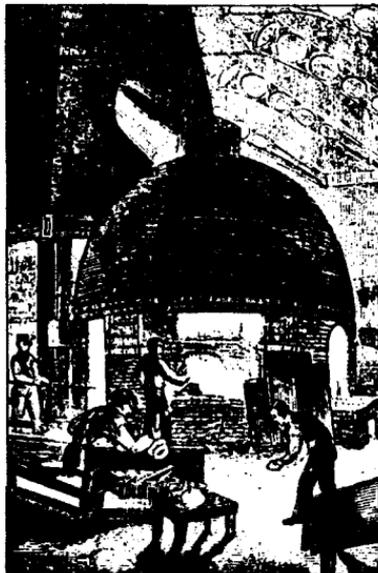
and the apprentices peer hopefully into the interior, but even when gold has melted into suspension the liquid remains clear. The fire is allowed to die down and all wait around the pot with bated breath. Slowly, slowly the glass cools until suddenly a roseate glow transfigures the watery liquid and it becomes deep ruby red.
